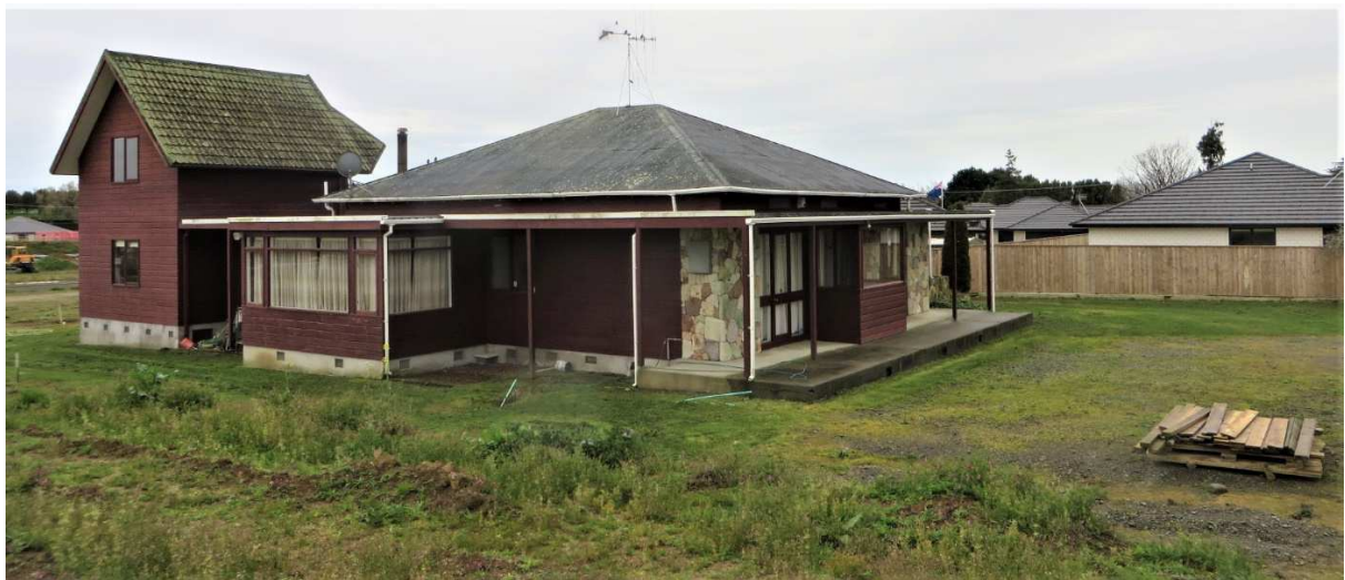
The iconically-clad homestead today, adrift within a housing development
