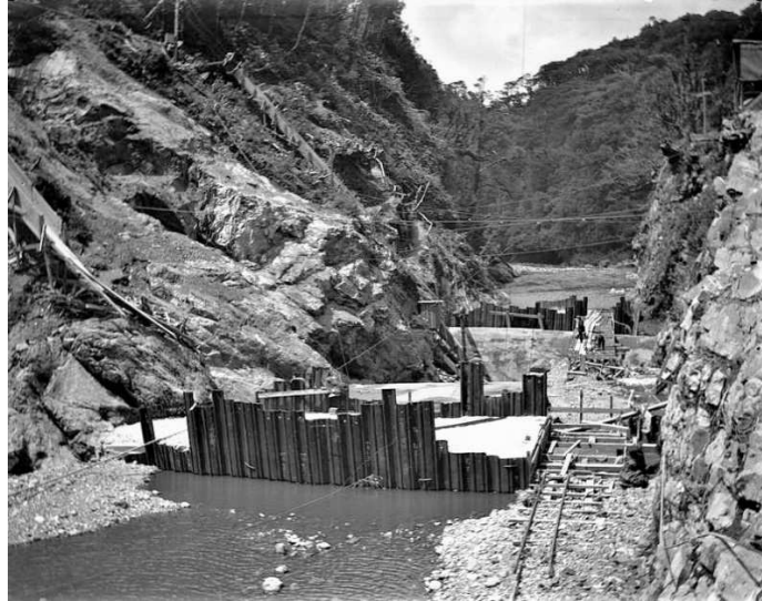
Mangahao construction photo taken by Leslie (PICRYL Public Domain Image)
